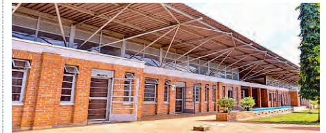
UNITE Kaliro Campus: String of Lecture Blocks
