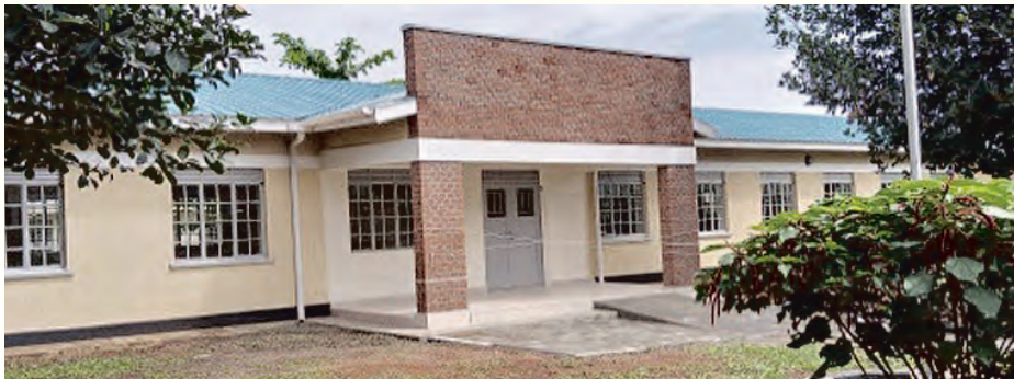
UNITE Main Campus: Start-up Headquarter Offices at Kitikifumba (Shimoni), Kira Municipality
